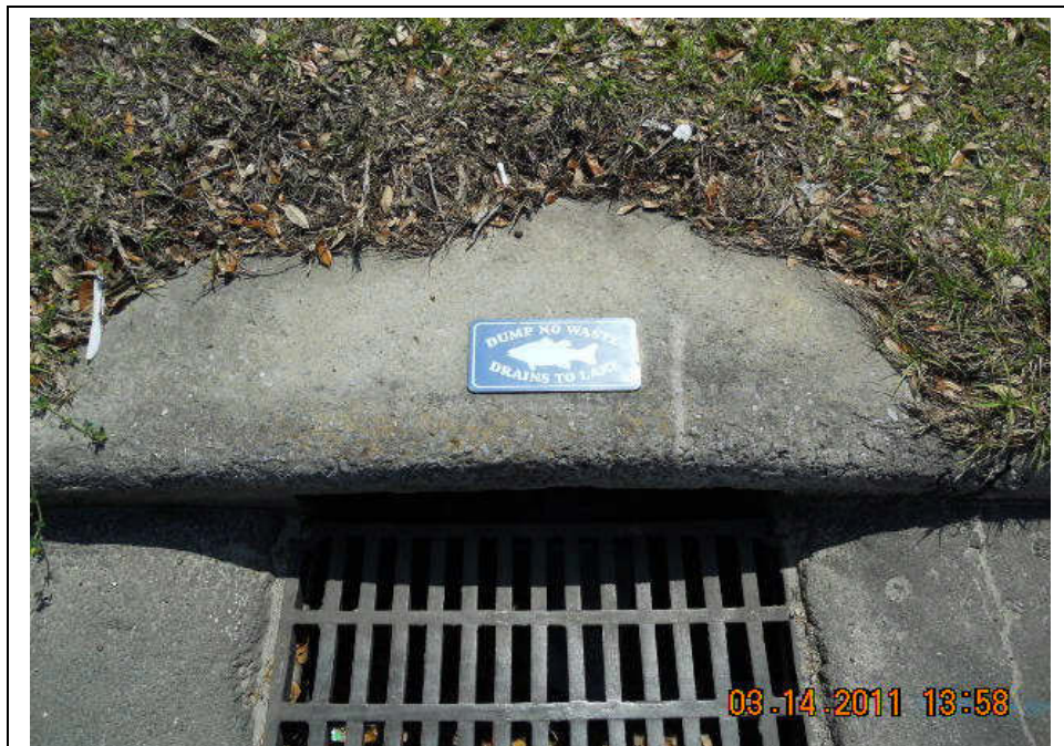
Photograph 8: View of storm water catch basin indicating stormwater drains to lake.
