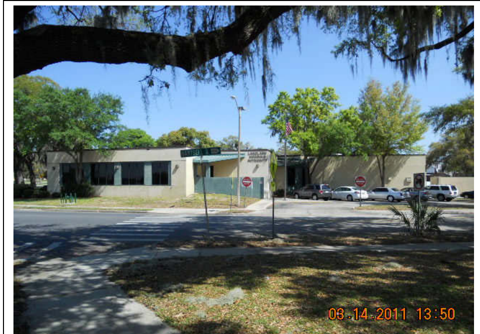
Photograph 3: View of the Central Office facility (430 Hartsell Avenue), facing east.
