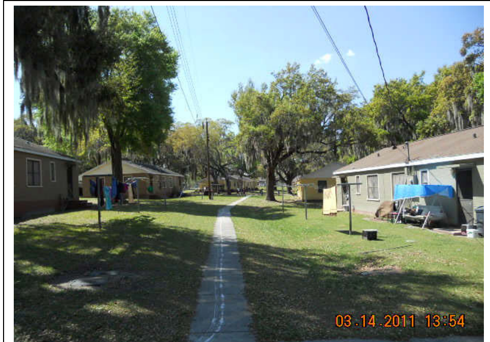
Photograph 7: View facing west across central portion of Subject Property.
