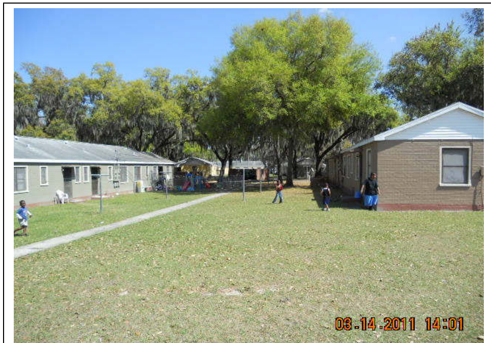
Photograph 12: View facing east across the central portion of the Subject Property.
