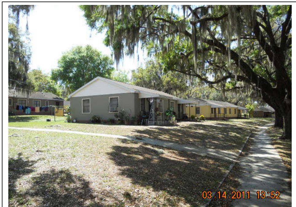
Photograph 4: View of apartments (typical).
