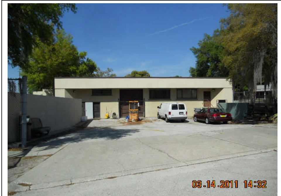
Photograph 25: View of southern elevation of Central Office.
