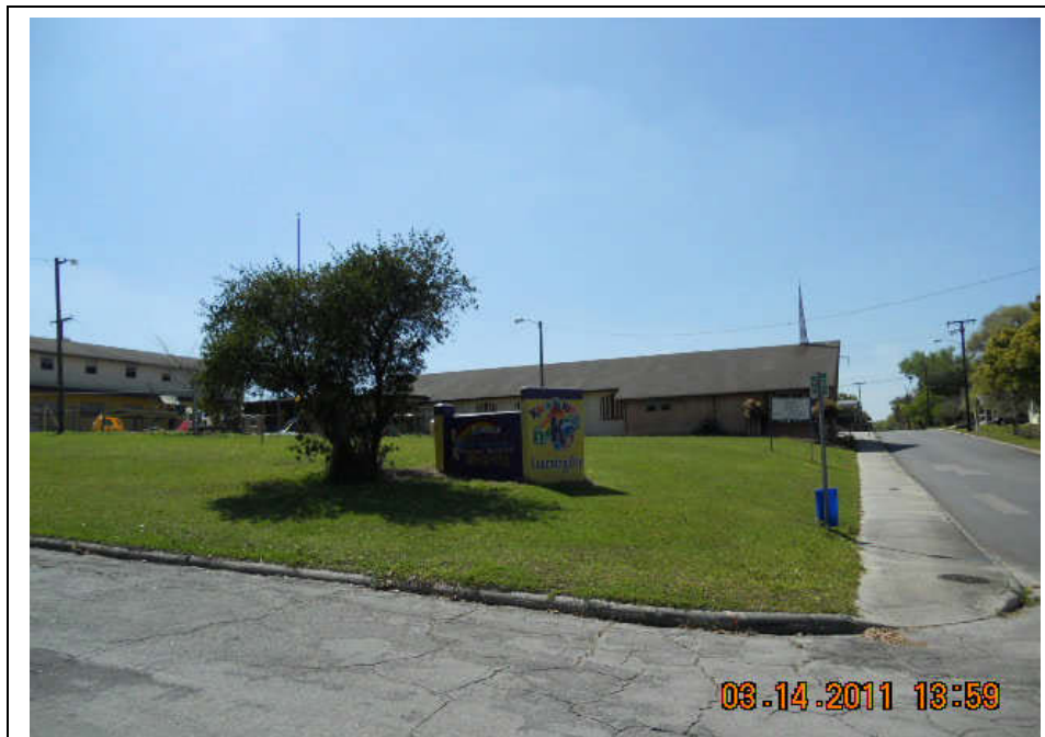
Photograph 10: View of daycare center adjacent west of the Subject Property.
