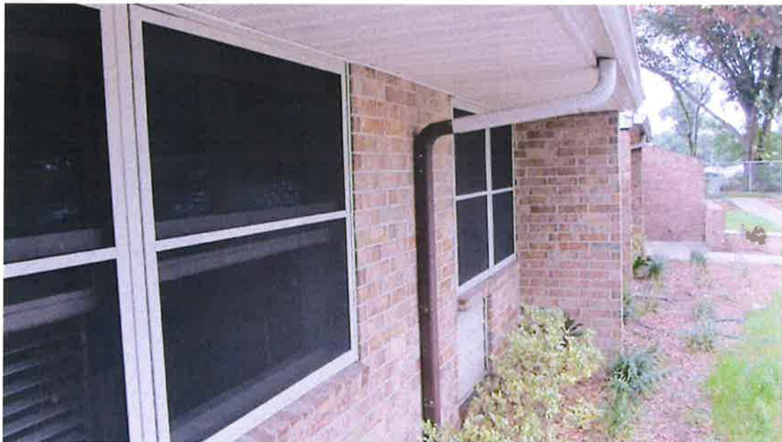
Photograph 6) – View looking north along the front elevation of Unit #19.
