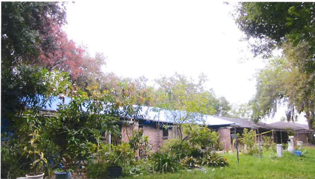
Photograph 4) – Rear (west) elevation.
