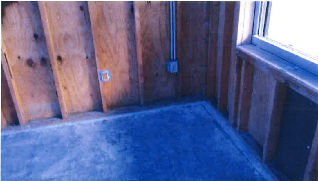
Photograph 39) – Interior view of the exterior load-bearing wall framing.
