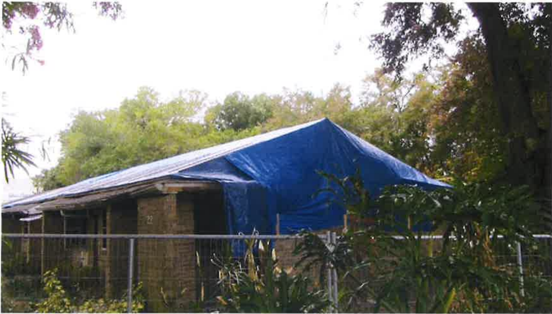
Photograph 3) – Right (north) elevation at Unit #22.
