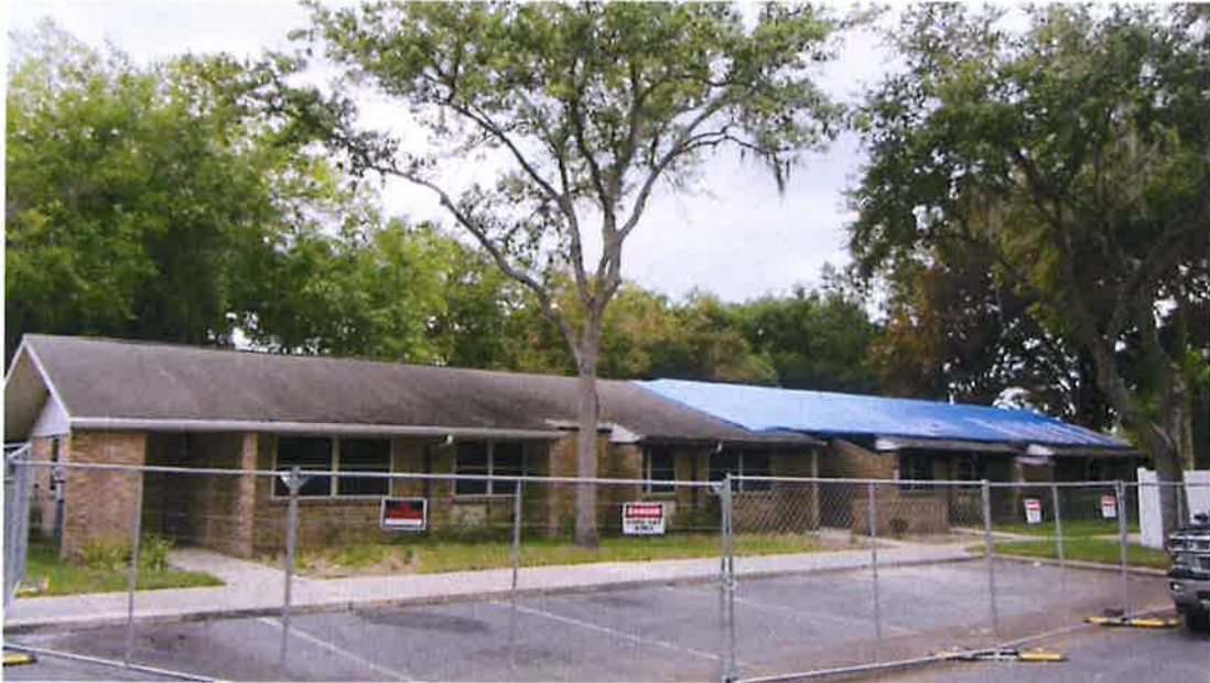
Photograph 1) – Front (east) elevation.
