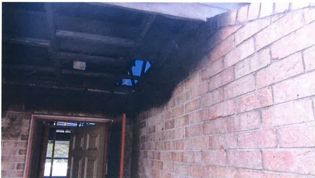
Photograph 32) – View looking west at the front entry foyer of Unit #20.
