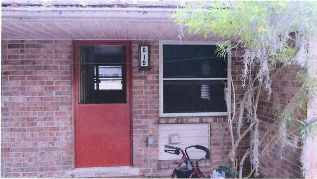
Photograph 9) – View looking east at the rear covered patio of Unit #19.
