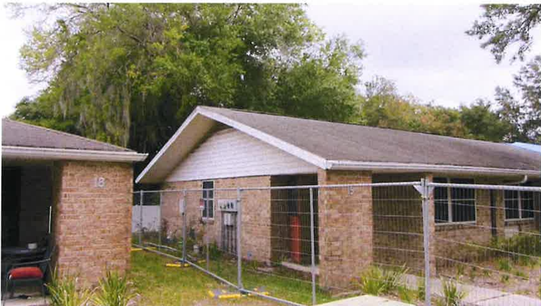
Photograph 2) – Left (south) elevation at Unit #19.
