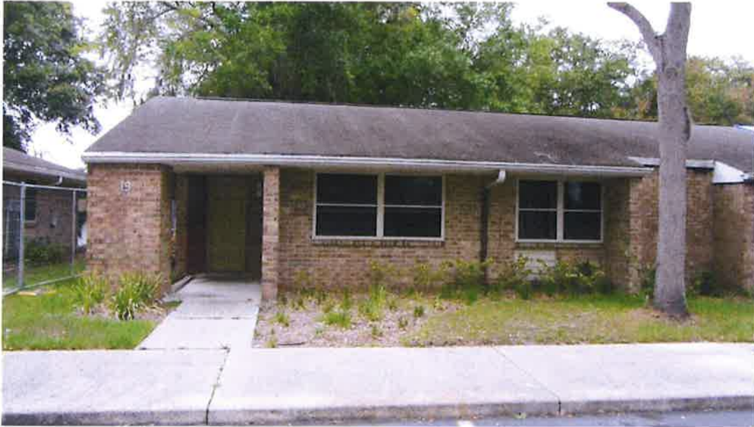
Photograph 5) – Exterior view of Unit #19.
