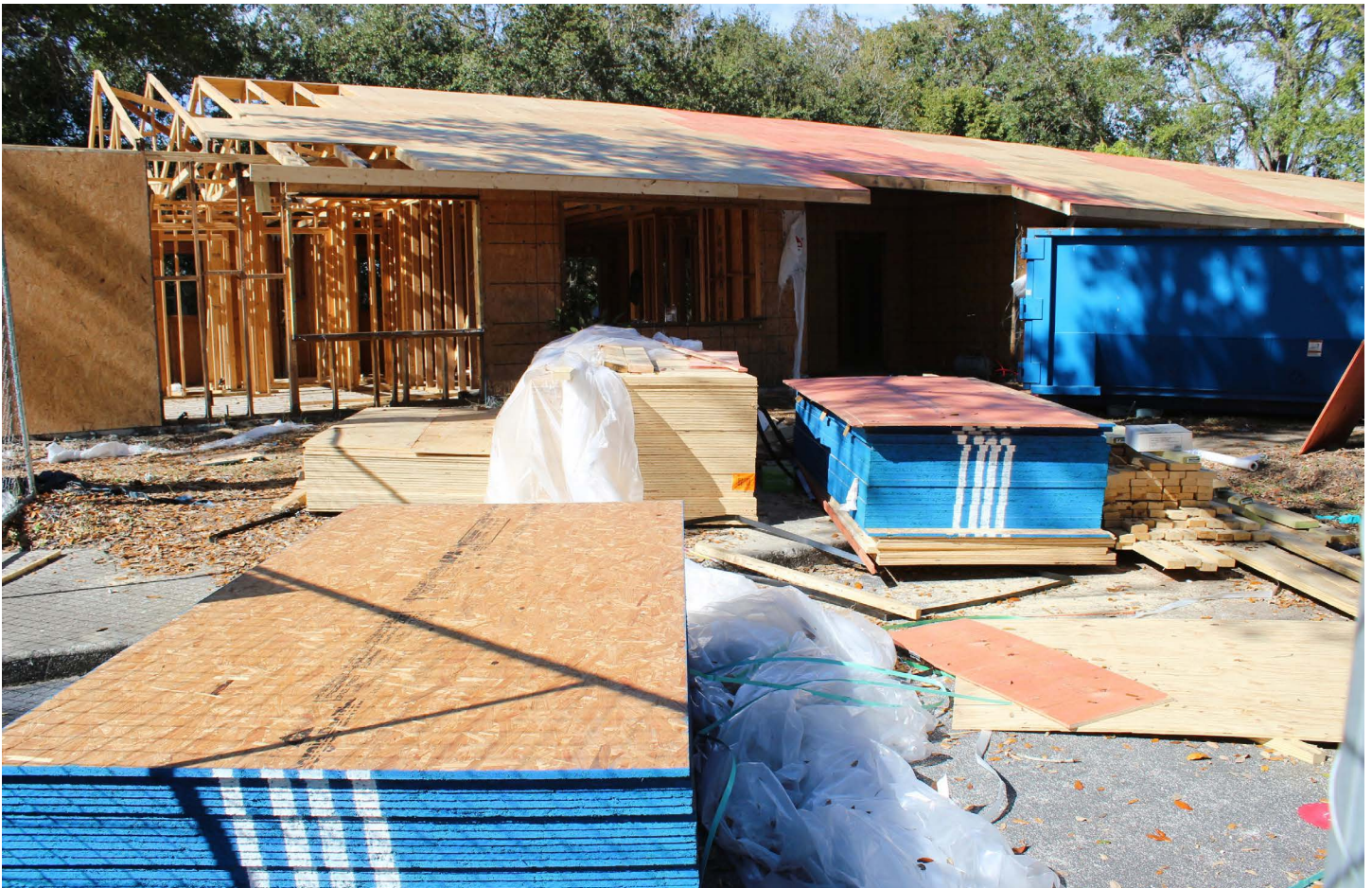
Four units being renovated at Cecil Gober Villas.
