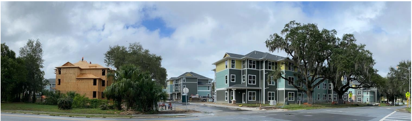
View of housing units along Hartsell Avenue
