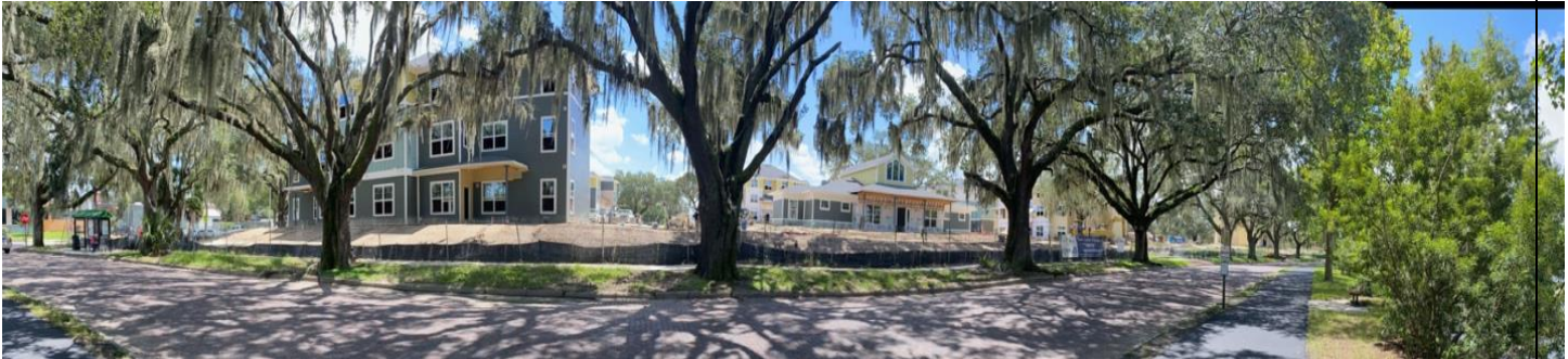
View of community center and housing units along Olive Street
