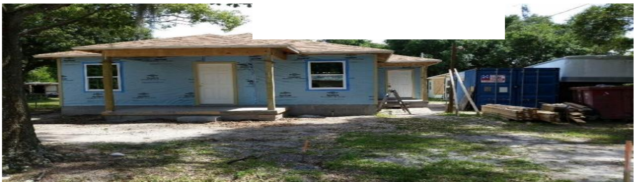
YouthBuild/Habitat project at Strawberry Lane in Lakeland
