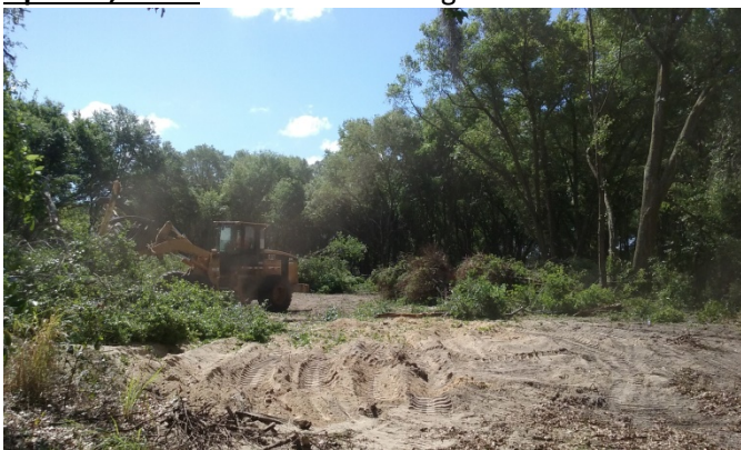
April 14, 2017: Additional clearing that occurred at the site.
