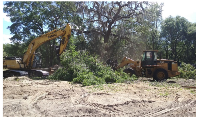
April 14, 2017: Continued clearing of site.
