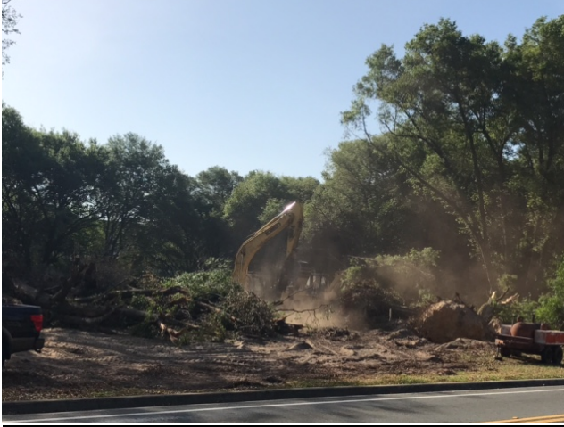
April 17, 2017: Continued clearing and grubbing.
