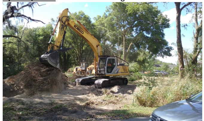
April 14, 2017: Continued clearing activities.
