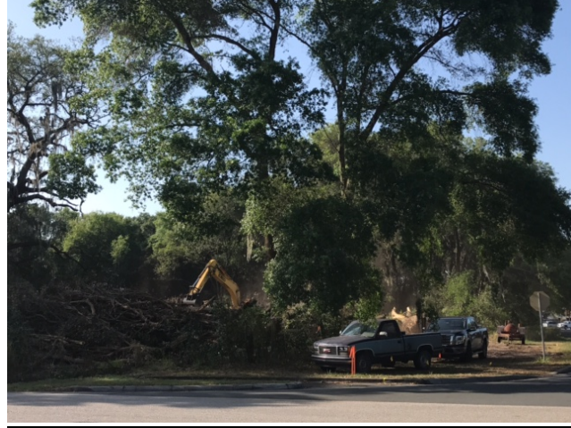
April 17, 2017: Another photograph of clearing and grubbing.
