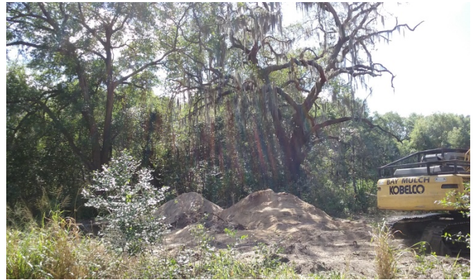
April 14, 2017: Picture of site contractor clearing trees.
