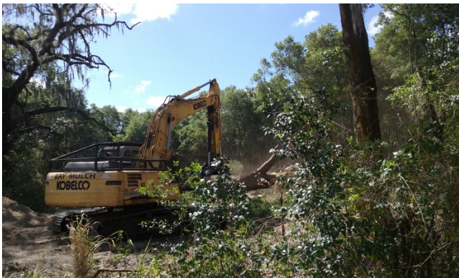
April 14, 2017: Continued clearing of site.
