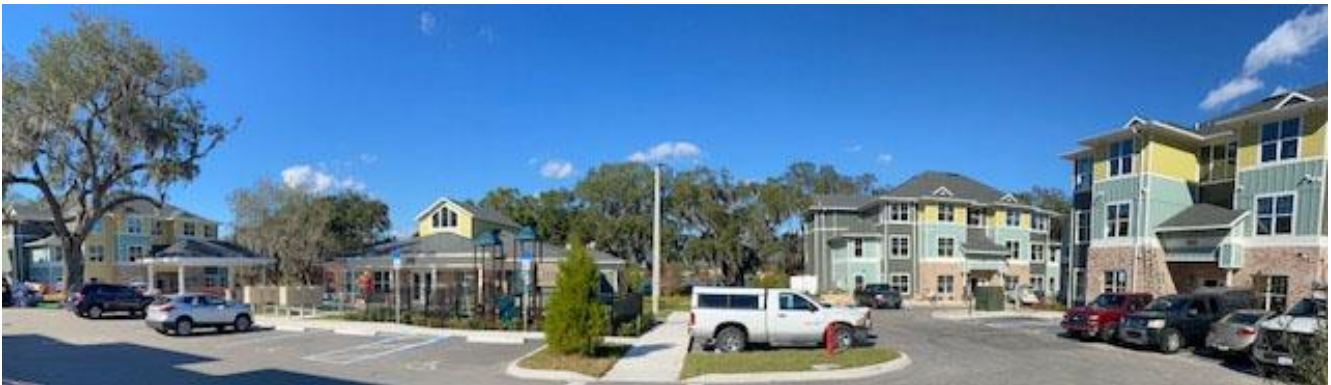
View of community center from parking lot.
