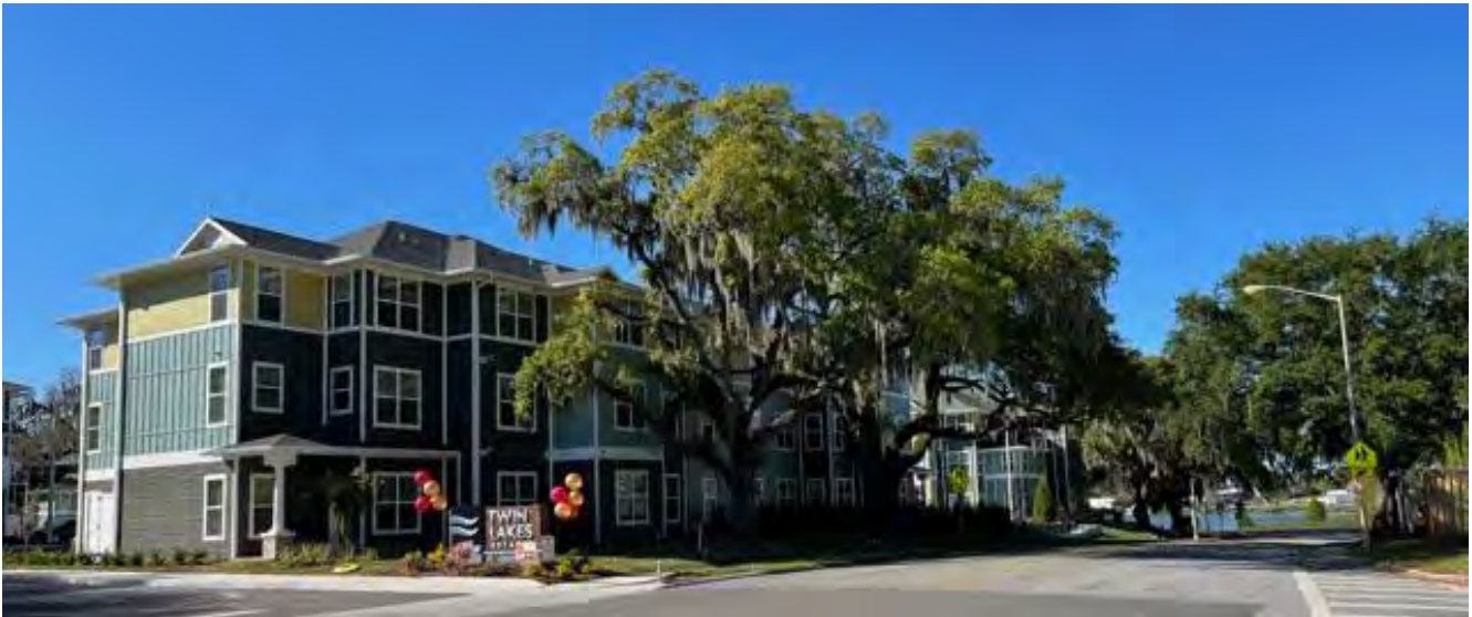
Entrance to the property off of Hartsell Avenue.
