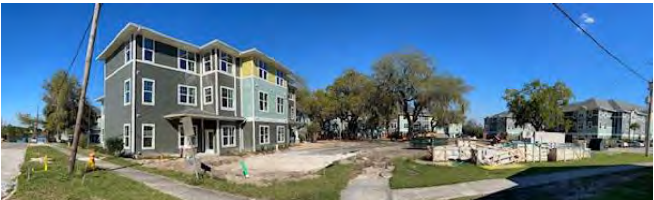
View of construction progress on the westside of the property.
