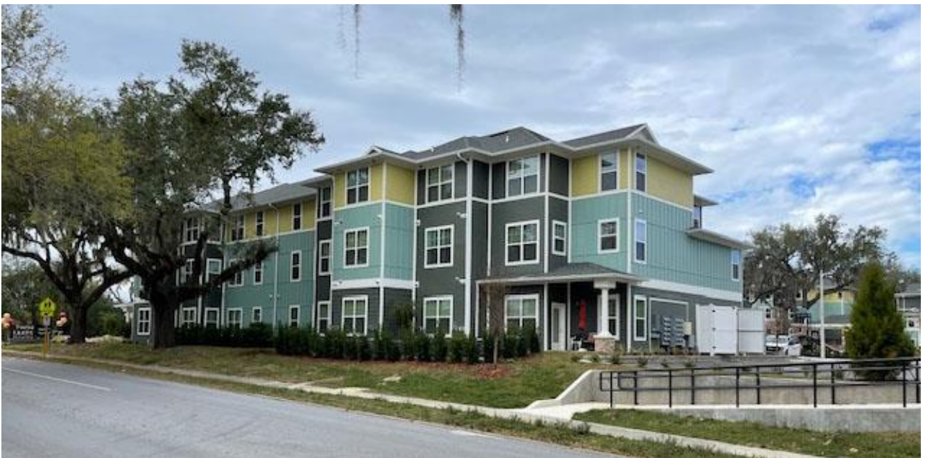
View of housing unit on Hartsell Avenue
