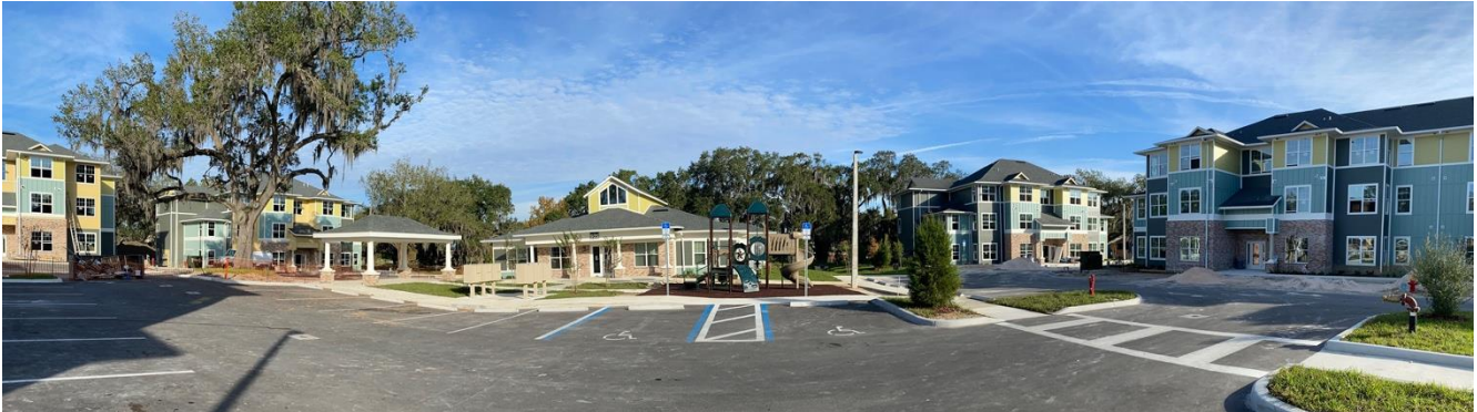
View of community center from parking lot.
