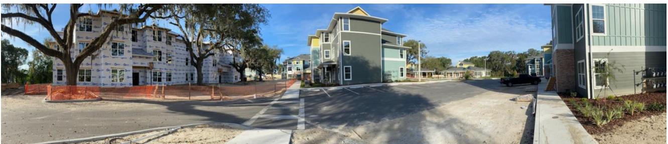
View of construction progress on southside of property.
