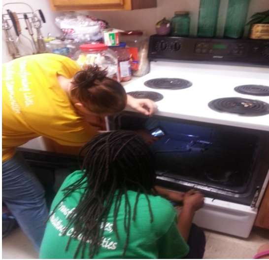
Participants help repair a stove
