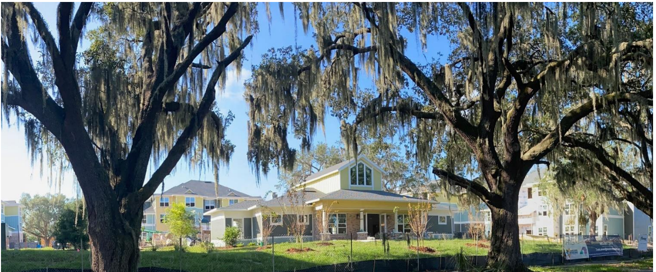
Closeup view of community center on Olive Street
